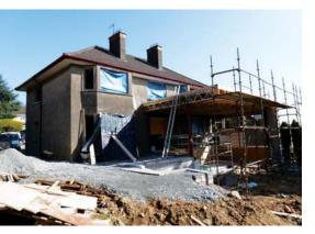
(above) As the living areas of the house were south-facing, an extensively glazed extension was built to make the most of the solar gains. The sloped garden facilitated in dropping the floor level, allowing the design team to increase the height of the extension; (p67, clockwise from top left) airtightness was achieved through a combination of OSB board and Siga tape; Knauf Earthwool insulation in the flat roof of the extension; an overhang provides summer shading.
